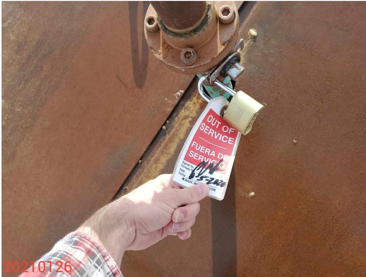
Photo 2: Continued from photo 1. Photo shows riser at valve can has been LO/TO
