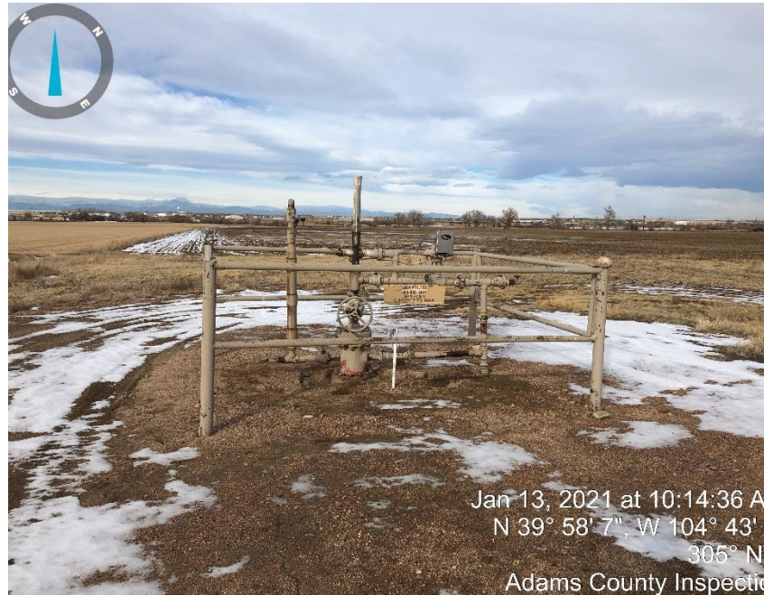
Photo #3 Well Head.
