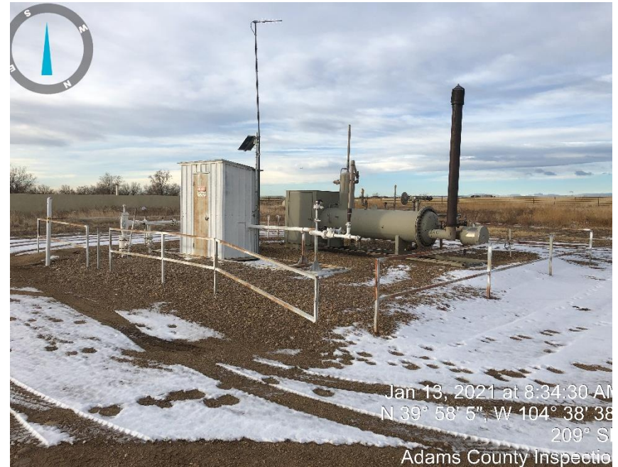
Photo #2 Separator & Meter.
