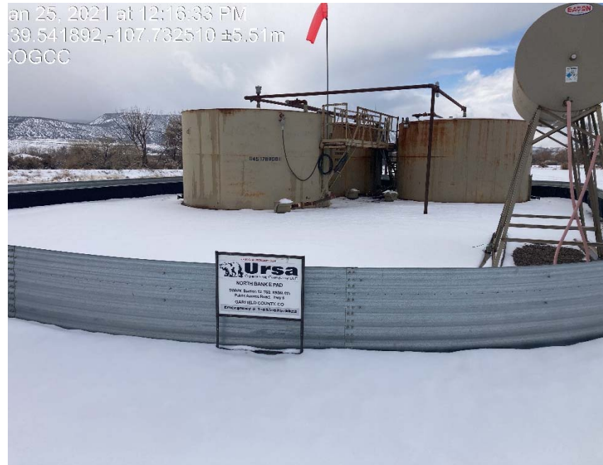
Location/Battery signage missing information
