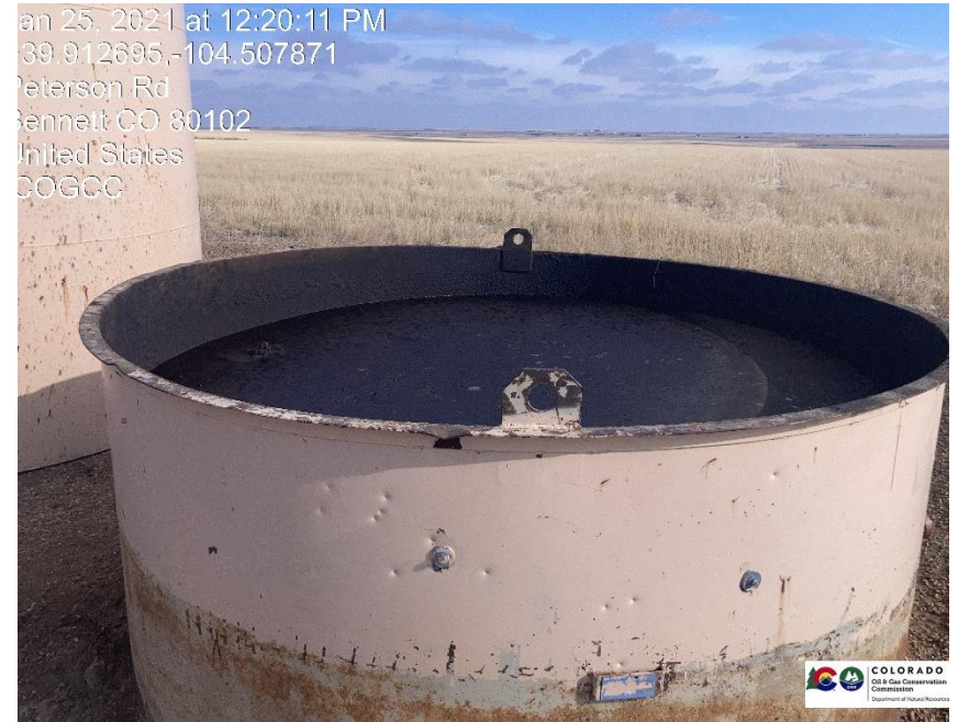
Pic 6 open top tank with no netting
