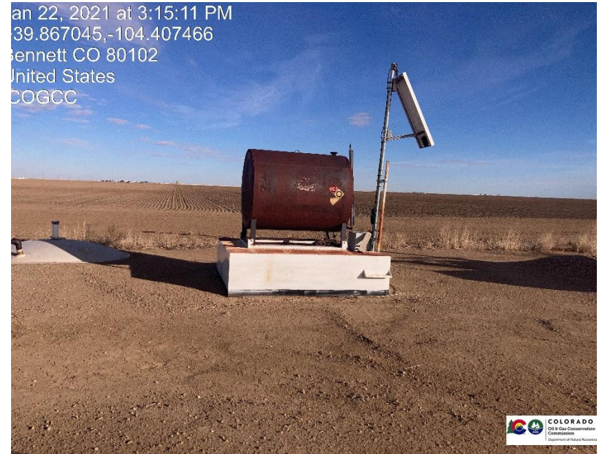
Pic 4 unused equipment on location
