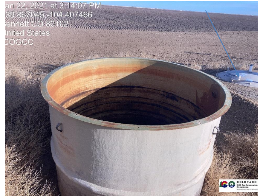
Pic 2 no wildlife protection on tank. Top sitting nest to tank
