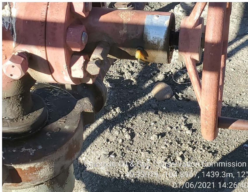
Master valve leak on 1/6/2021
