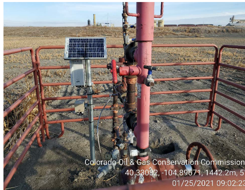
Lubricator leak on 1/25/2021
