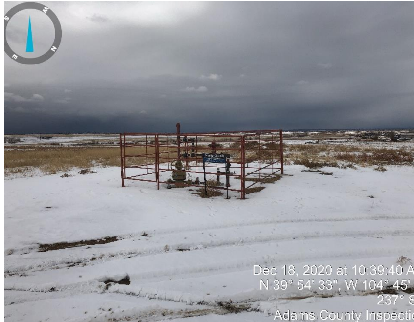
Photo #3 Well Head.
