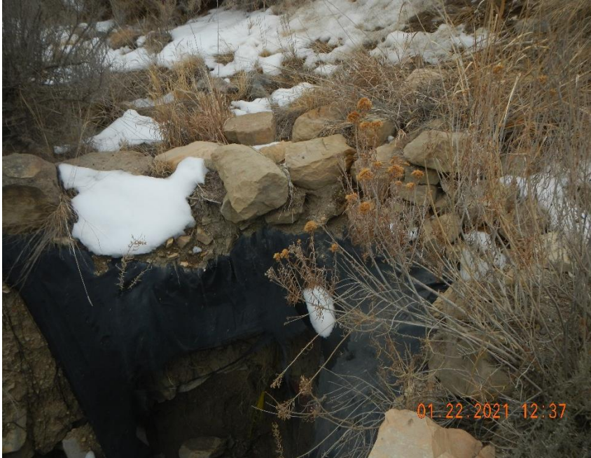
Erosion damage from culvert outlet.
