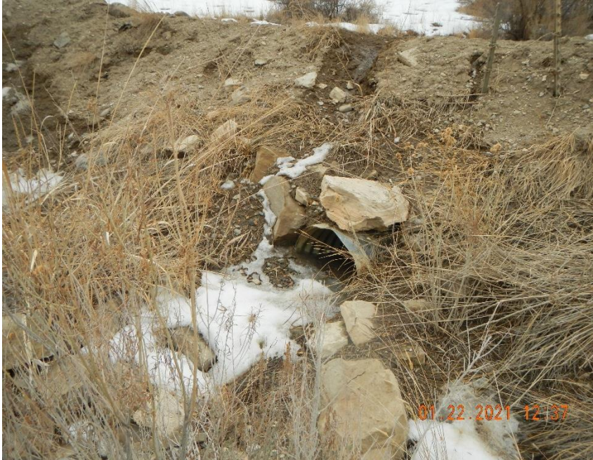
Sediment build up in culvert outlet.
