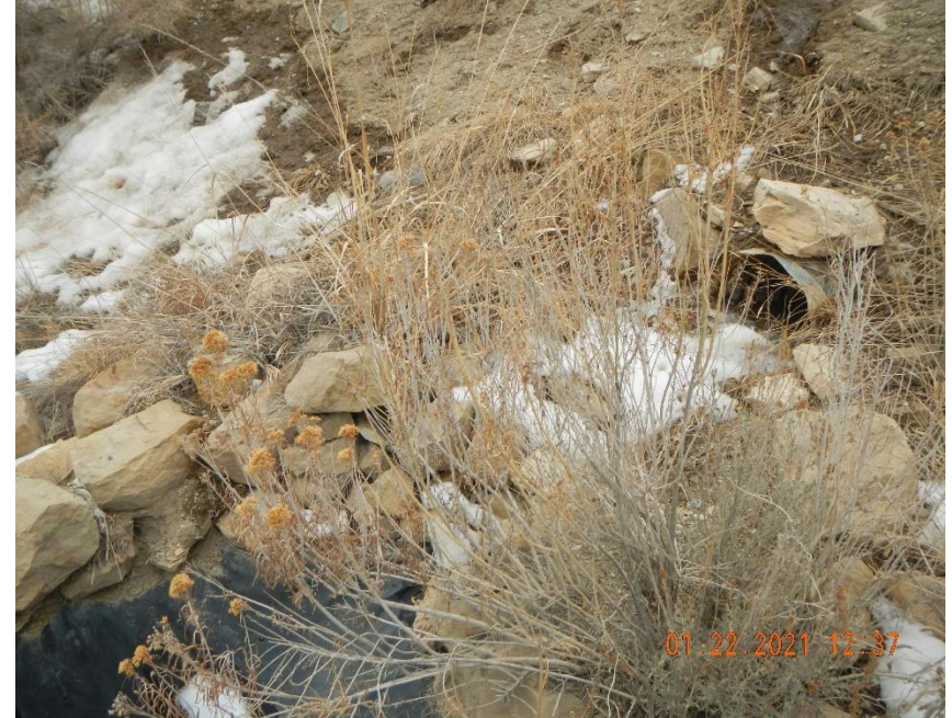
Erosion damage from culvert outlet.
