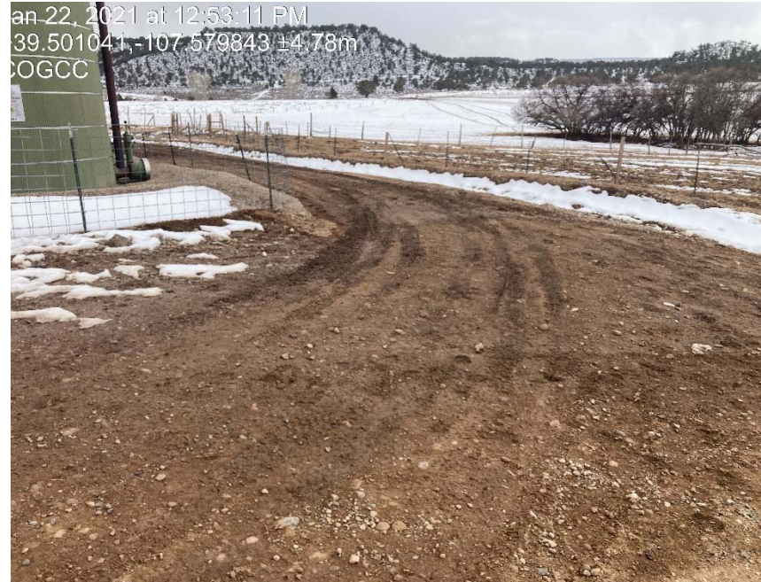
Lack of stabilization/Entrance/No evidence of tracking control BMP's
