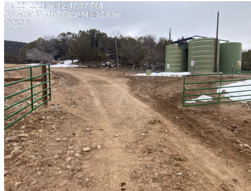
Entrance/No evidence of tracking control BMP's
