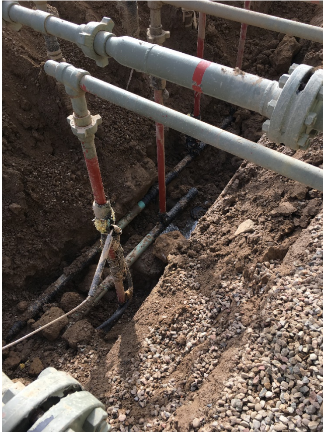
2" carbon steel dump line, release point at tee
