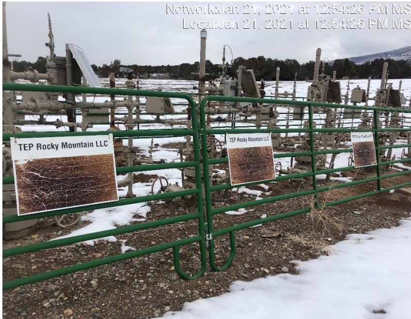
Photo #2686 Multiple wellhead signs weathered and not legible.
