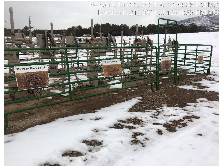
Phot #2687 Multiple wellhead signs weathered and not legible.
