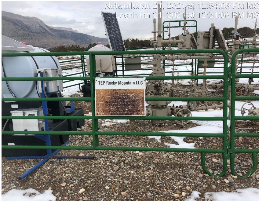
Photo #2684 Multiple wellhead signs weathered and not legible.
