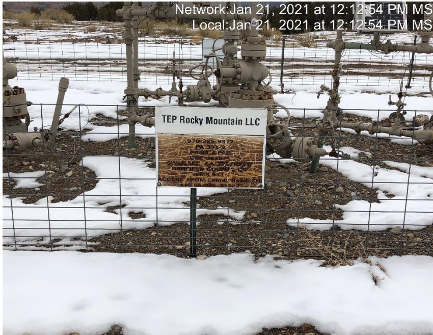
Photo #2679 Multiple wellhead signs weathered and not legible.
