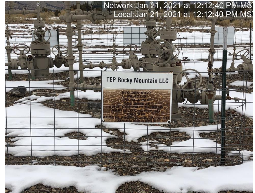
Photo #2678 Multiple wellhead signs weathered and not legible.
