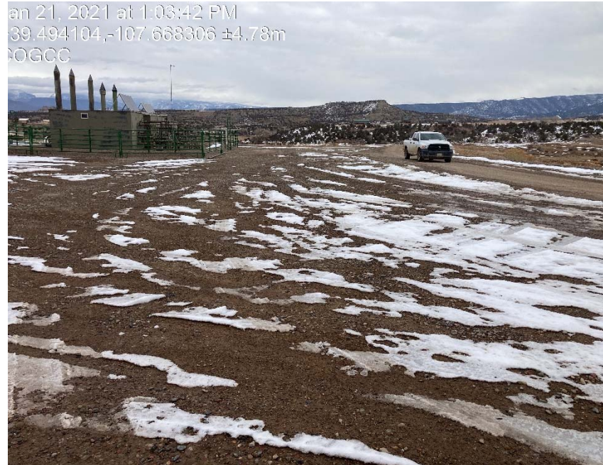
Entrance/no evidence of tracking controls/lack of stabilization
