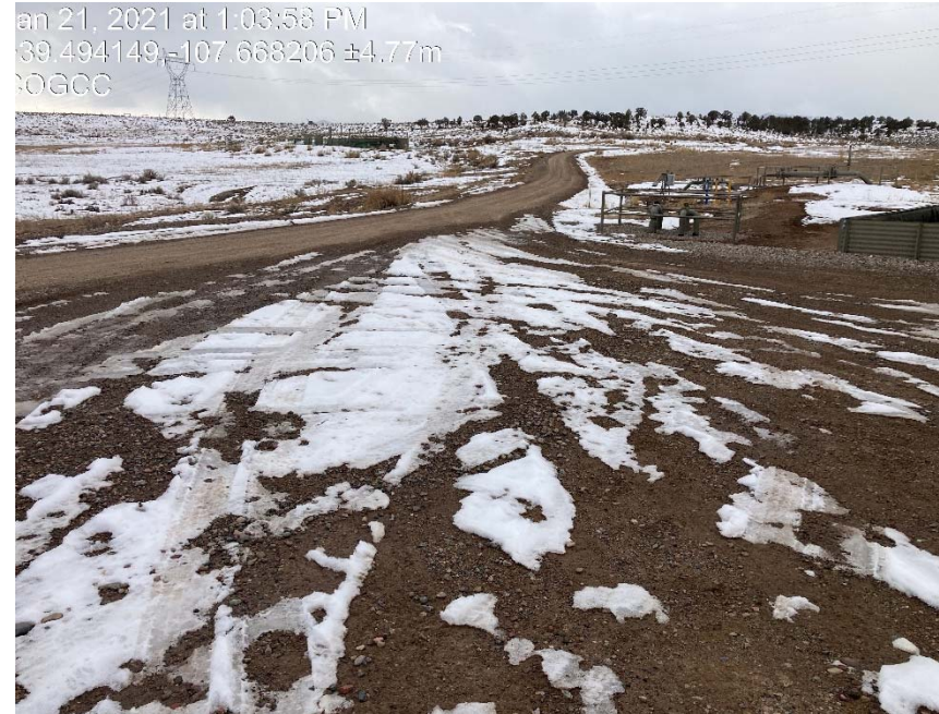
Entrance/no evidence of tracking controls/lack of stabilization
