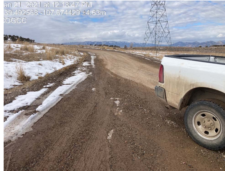
Entrance/no evidence of tracking controls
