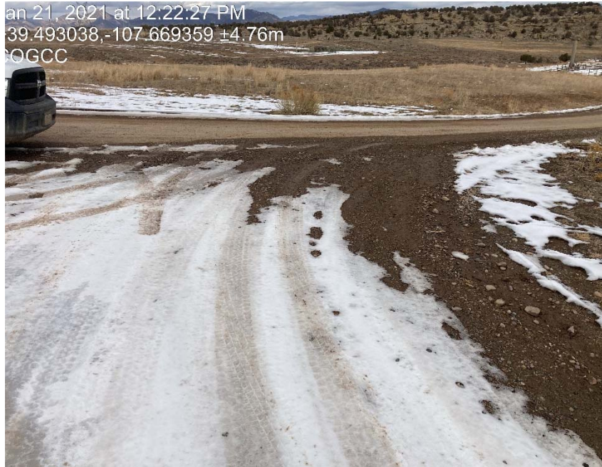
Entrance/no evidence of tracking controls
