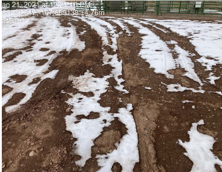
Lack of stabilization
