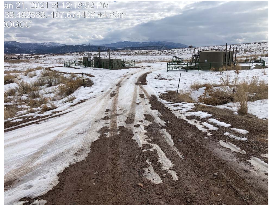
Lack of stabilization/entrance/no evidence of tracking controls
