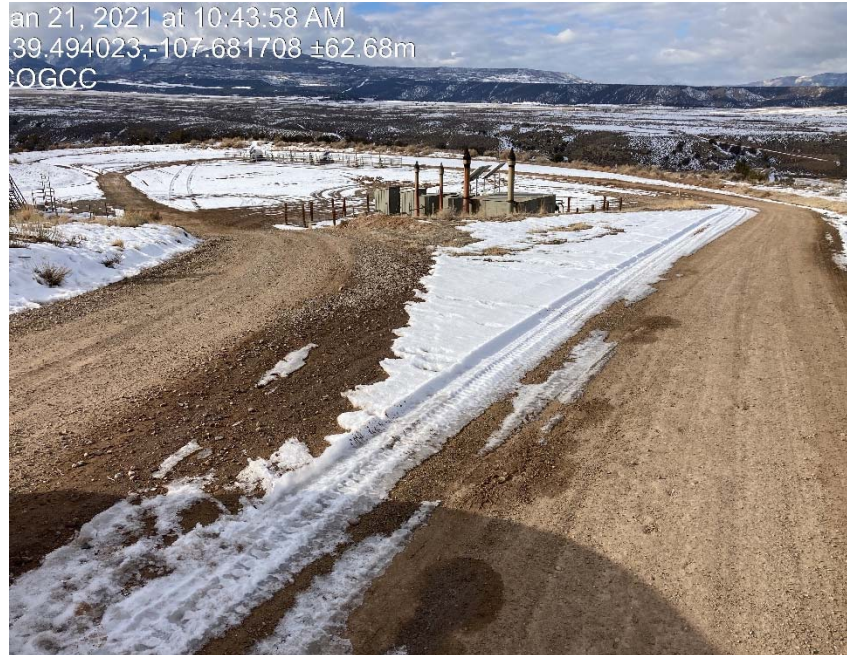
Lack of stabilization/entrance/no evidence of tracking BMP's
