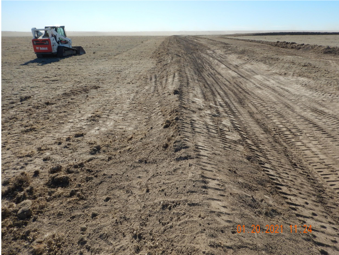
Photo 6. Photo taken from the eastern location, facing South. Photo illustrates the ditch and berm BMP, which has been installed around the entire perimeter of location.
