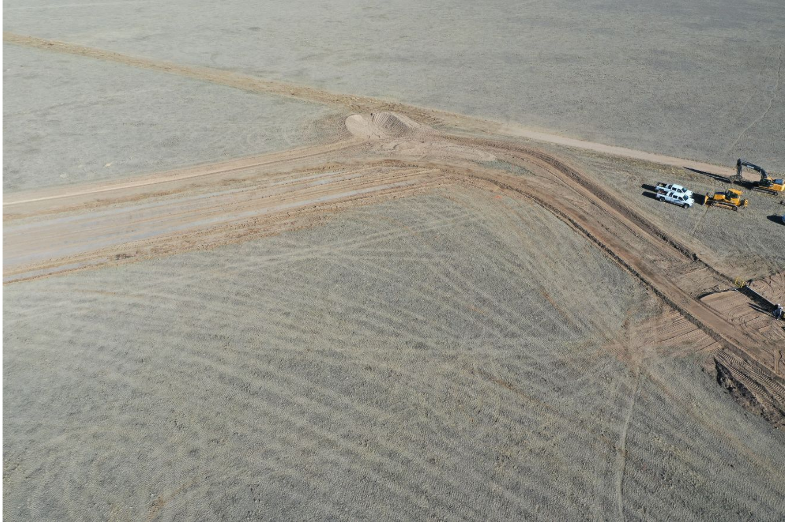
Photo 2. Drone aerial imagery illustrates the northeastern location, facing Northeast. Photo illustrates the ditch and berm BMP, and a sediment trap being completed.
