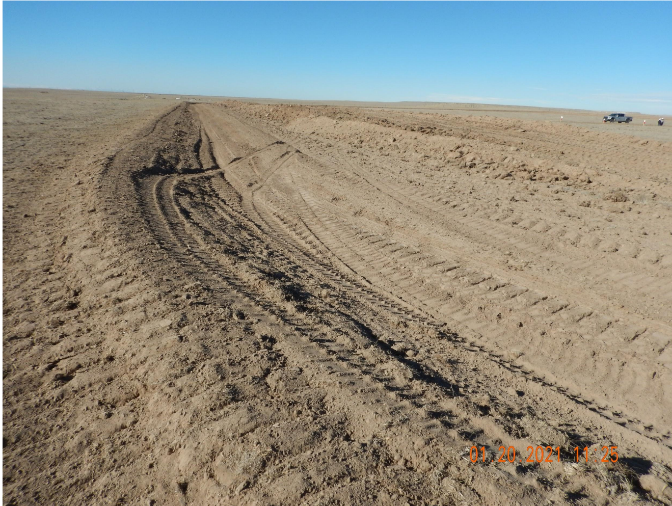
Photo 7. Photo taken from the southern location, facing West. Photo illustrates the ditch and berm BMP and the topsoil stockpile.
