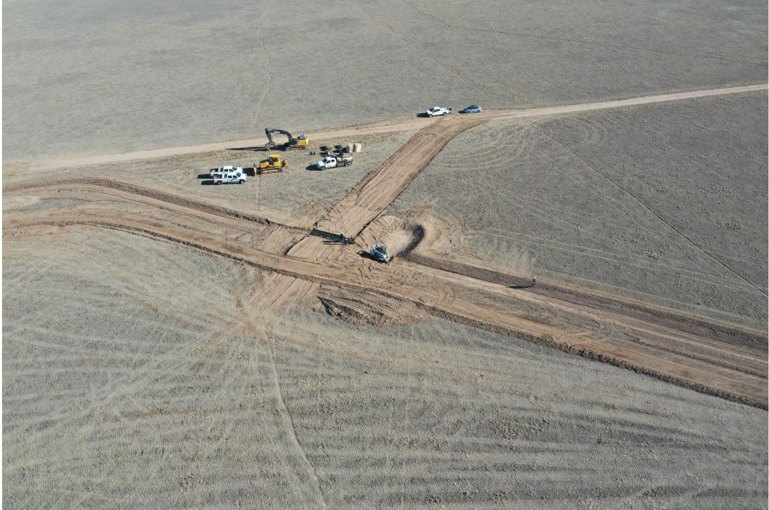
Photo 1. Drone aerial imagery illustrates the eastern location, facing East. Photo illustrates the new access road, ditch and berm BMP, and a sediment trap being completed.
