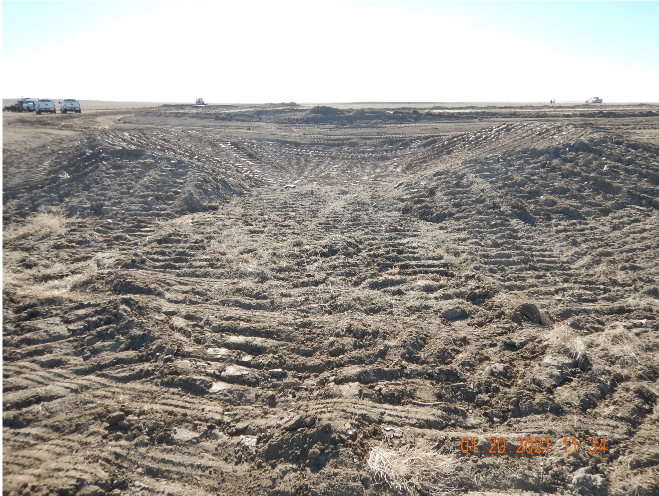
Photo 8. Photo taken from the northeastern location, facing South. Photo illustrates a sediment trap being completed. Rip-rap material was delivered for the tracking pad and sediment trap outlets.
