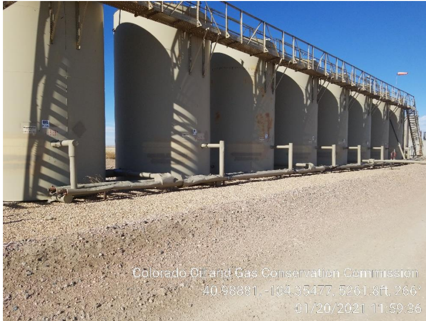
Photo 3 – Tank Battery
