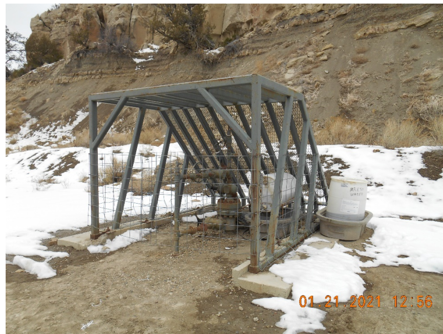
Wellhead with fencing. Secondary containment of chemicals.
