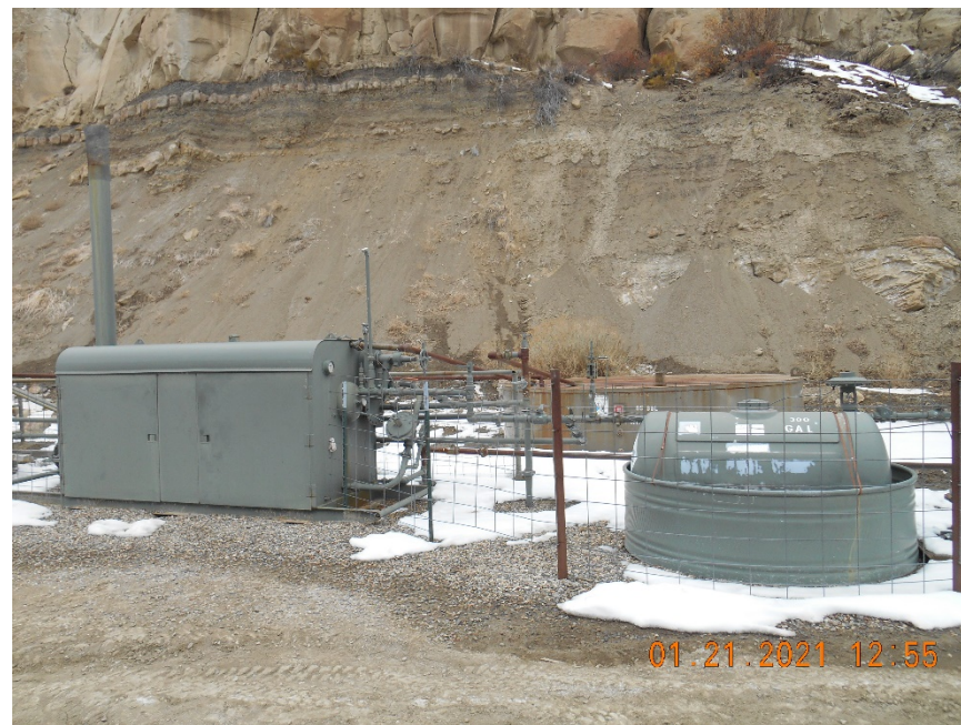
Separator with secondary containment of chemicals.
