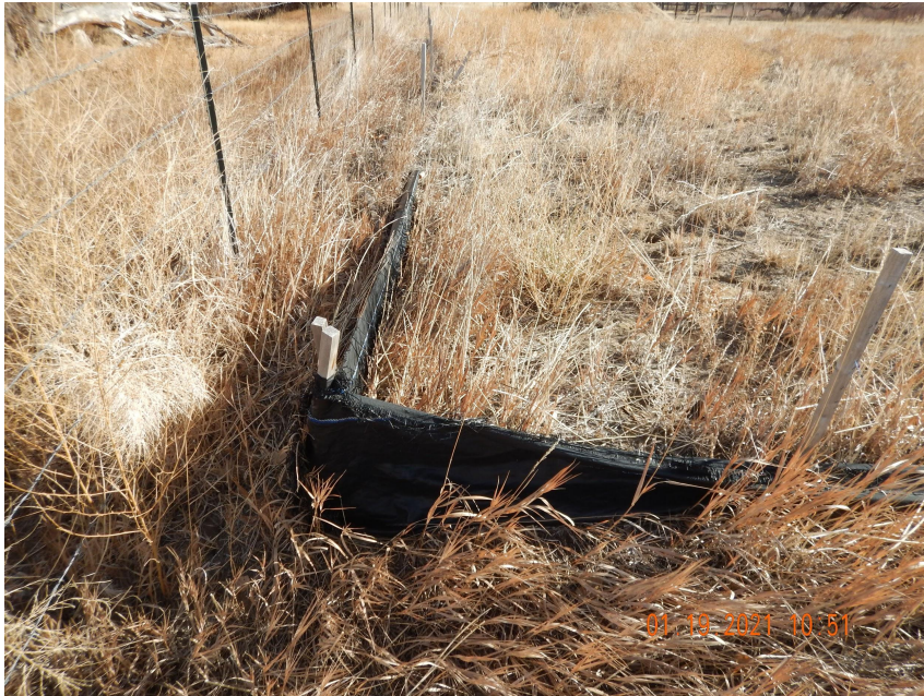
Photo 7. Photo taken from the northwestern perimeter of location, facing East. Photo illustrates the silt fence is no longer in proper functioning condition.
