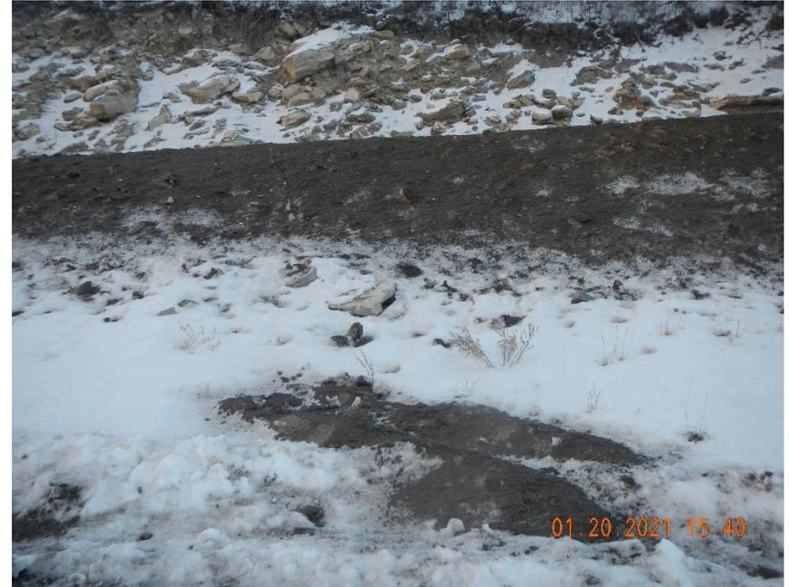
**Main road passes by location cutslope, sediment is moving from road onto cutslope.**
