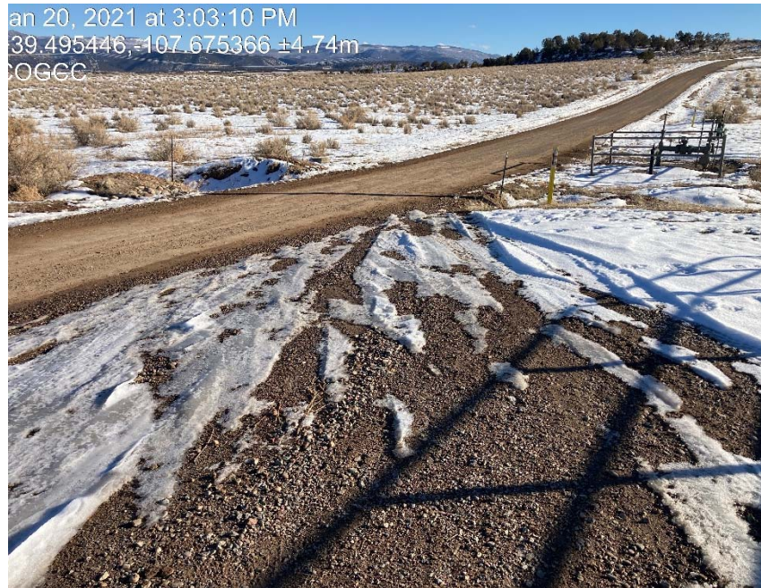
Entrance to separators/tank battery No evidence of tracking controls
