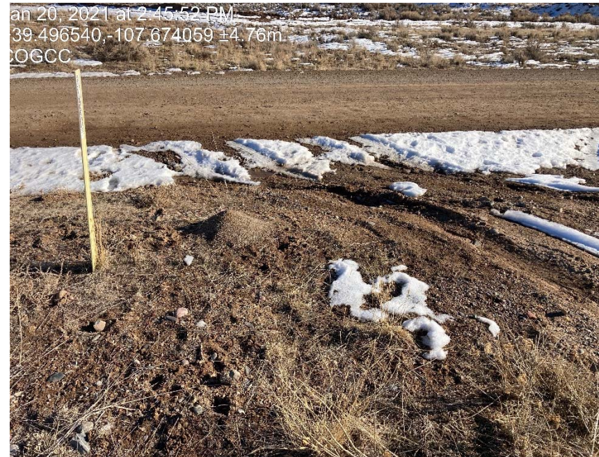
Entrance to well head/lack of stabilization/No evidence of tracking controls
