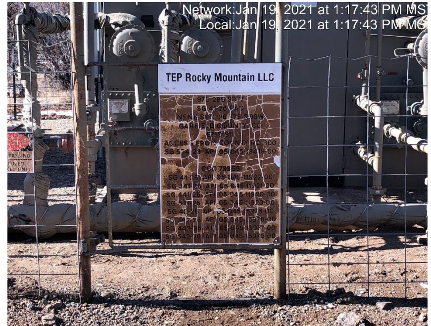
Photo #2655 Battery sign is weathered and not legible.
