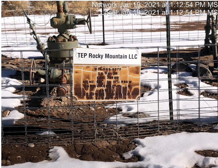
Photo #2651 Multiple wellhead signs weathered and not legible.
