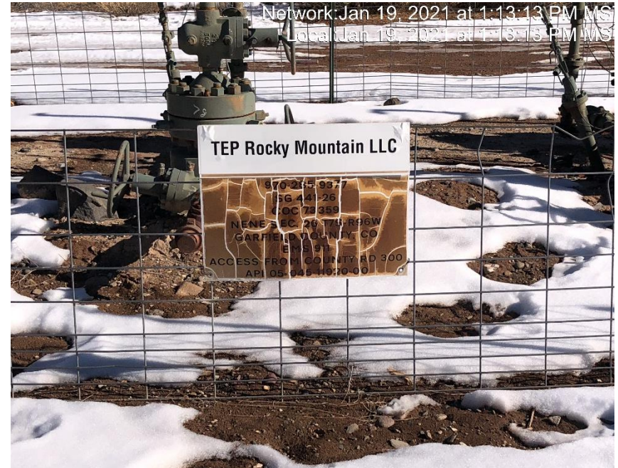
Photo #2652 Multiple wellhead signs weathered and not legible.
