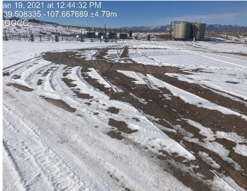
Location shows lack of stabilization/entrance/no evidence of tracking controls
