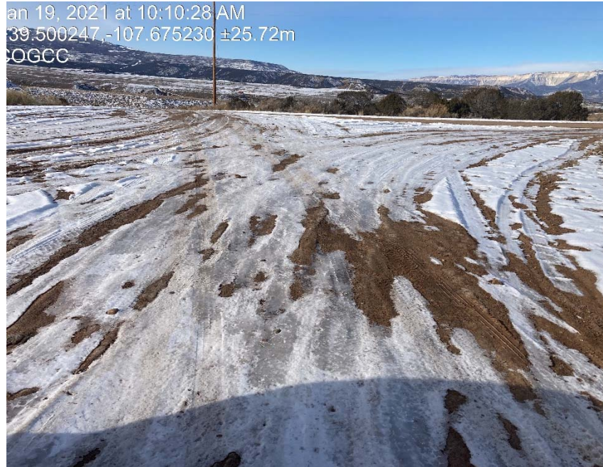
Location shows lack of stabilization/entrance
