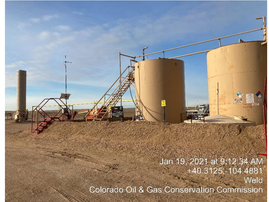
Photo #2 Tank Battery
