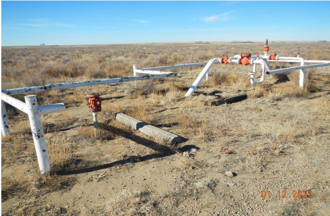
Photo 2. Pipe risers have not been removed at the west side of the location.
