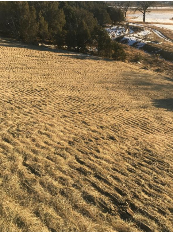
Photo of southwest portion of fill slope after recontour as near as practicable, seeding, mulching and crimping.
