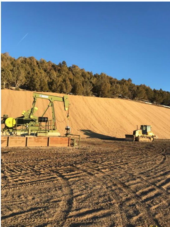
Photo of south end of cut slope after recontour as near as practicable, seeding, mulching and installation of 100% biodegradable ECB.
