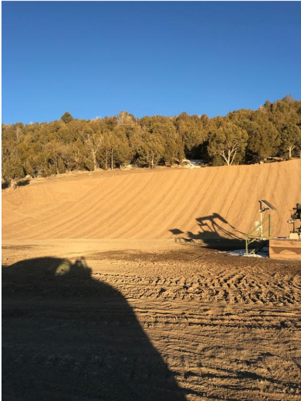
Photo of North end of cut slope after soils from fill slope were moved into cut to reduce slope and increase potential for seed germination and vegetation establishment.
