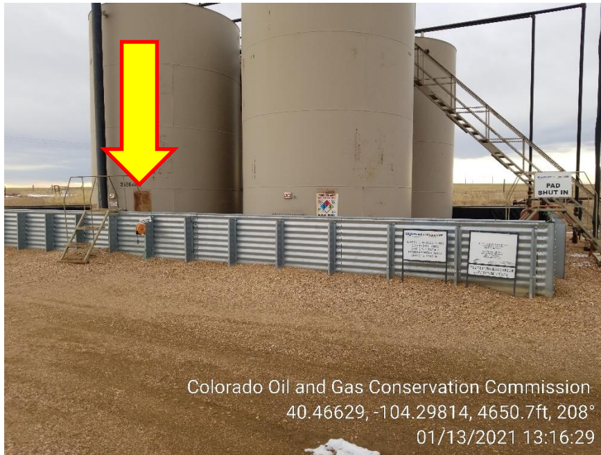
Photo 3 – Tank Battery, Crude Oil Tank missing Labels
