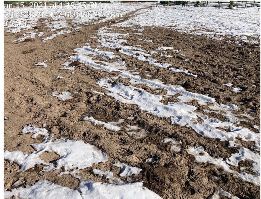
Lack of stabilization/rutting is present
