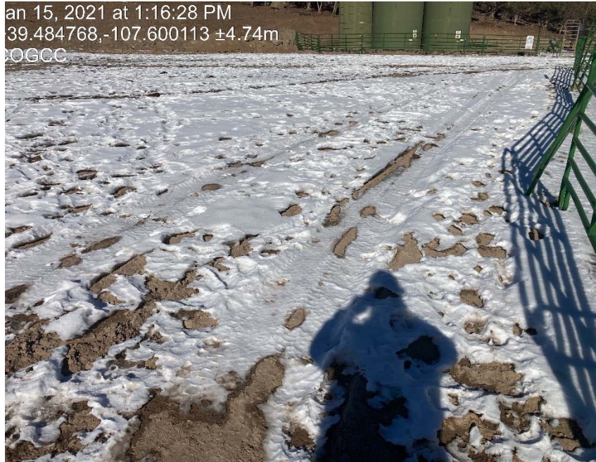
Lack of stabilization/rutting is present
