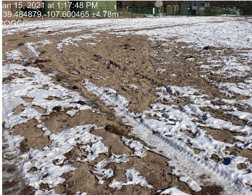
Lack of stabilization/rutting is present
