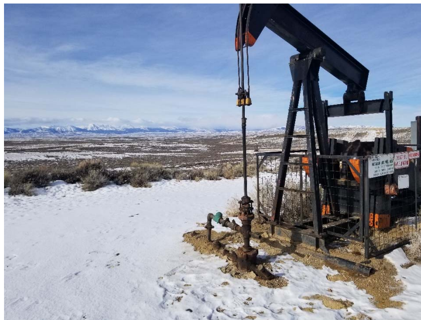
Photo 3. No bradenhead access apparent.
