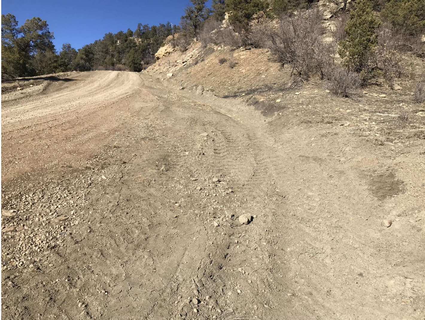
PHOTO 1: THE BAR DITCH WAS RECONFIGURED TO ELIMINATE THE EROSION AND THE SOIL WAS COMPACTED WITH THE TIRE OF THE BACKHOE FOR STABILIZATION.
