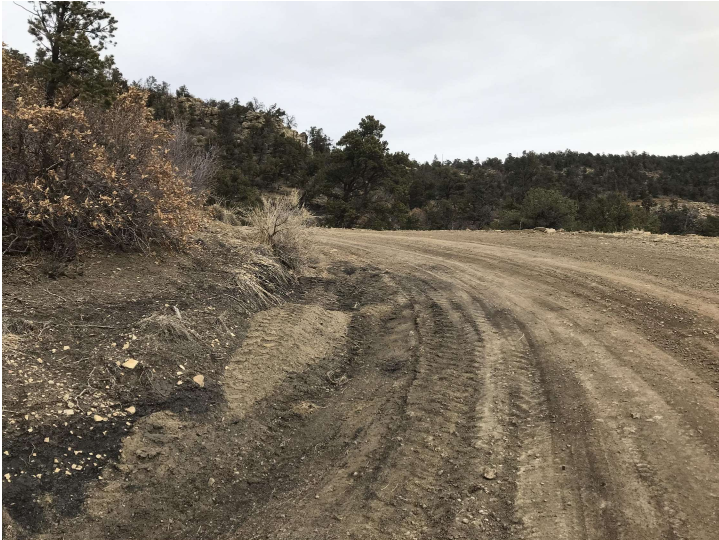
PHOTO 2: THE BAR DITCH WAS RECONFIGURED TO ELIMINATE THE EROSION AND THE SOIL WAS COMPACTED WITH THE TIRE OF THE BACKHOE FOR STABILIZATION.
