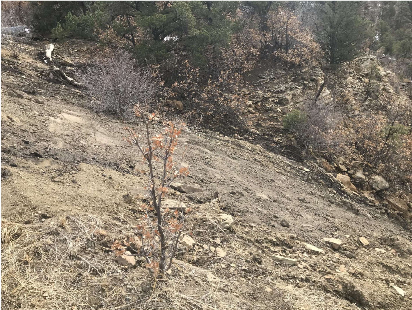
PHOTO 5: THE EROSION ON THE ACCESS ROAD FILL SLOPE WAS BACK FILLED AND THE SOIL WAS COMPACTED.
