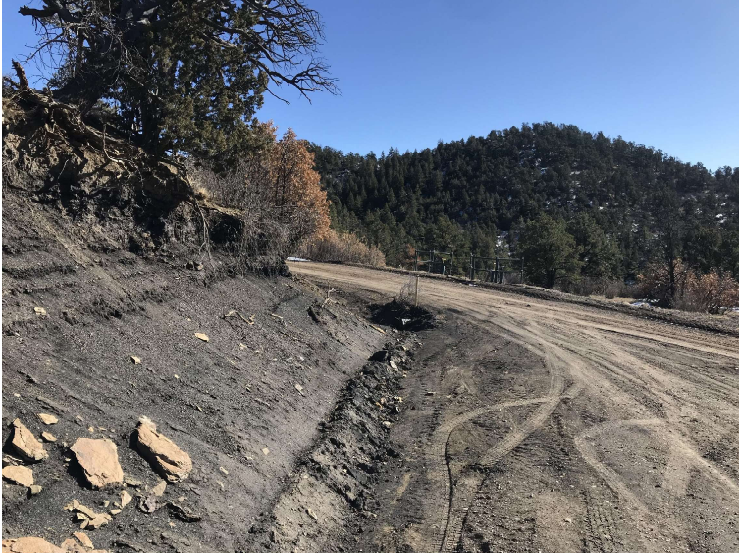
PHOTO 4: THE BAR DITCH WAS DOMINATED TO RECEIVE STORMWATER RUN OFF WHICH IS DIRECTED TO THE CULVERT INLET ON THE MAIN ROAD.
