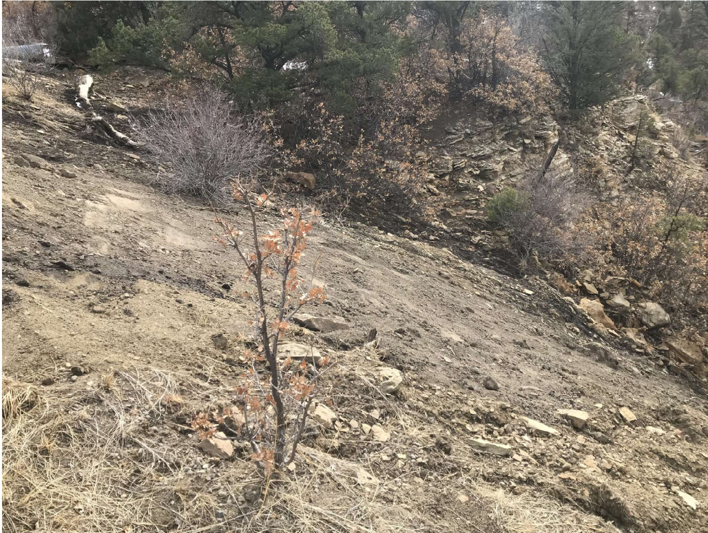
PHOTO 2: THE EROSION ON THE ACCESS ROAD FILL SLOPE WAS BACK FILLED AND THE SOIL WAS COMPACTED.
