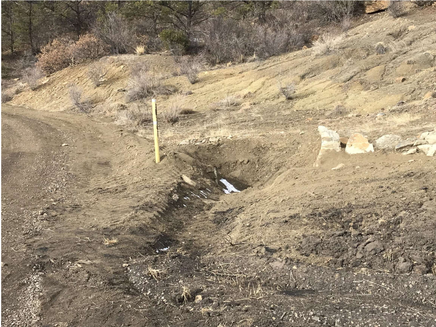
PHOTO 4: THE BELL HOLE WAS DOMINATED TO RECEIVE STORMWATER
