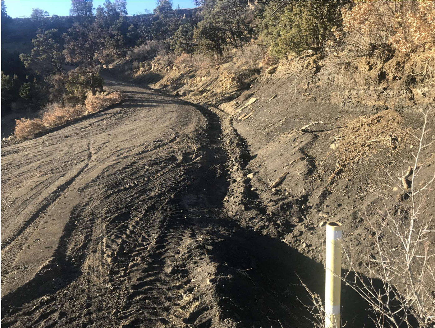
PHOTO 1: THE BAR DITCH WAS DOMINATED TO RECEIVE STORMWATER RUN OFF FROM THE UPLAND WATER SHED WHICH IS DIRECTED TO THE DOWN GRADIENT CULVERT INLET.
