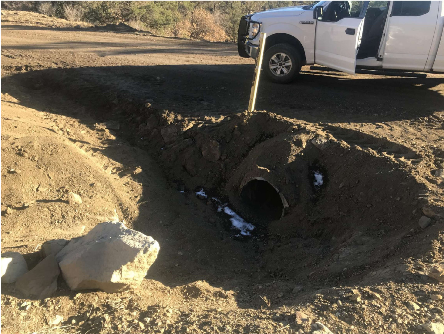
PHOTO 3: THE SEDIMENT ACCUMULATION WAS REMOVED FROM THE CULVERT INLET
