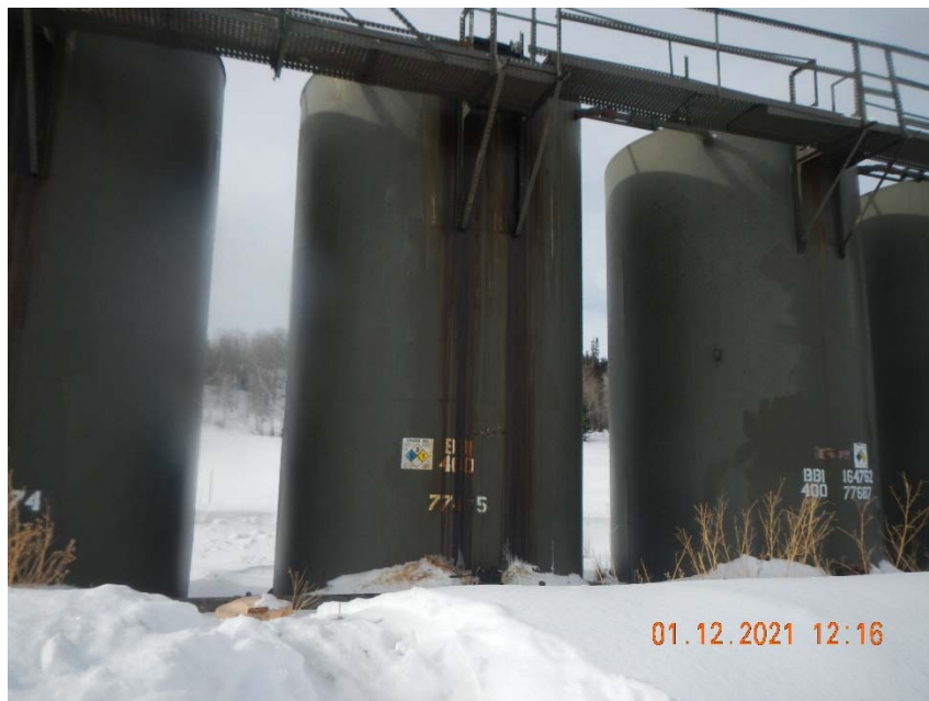
Photo 3. Staining from apparent overflow.
