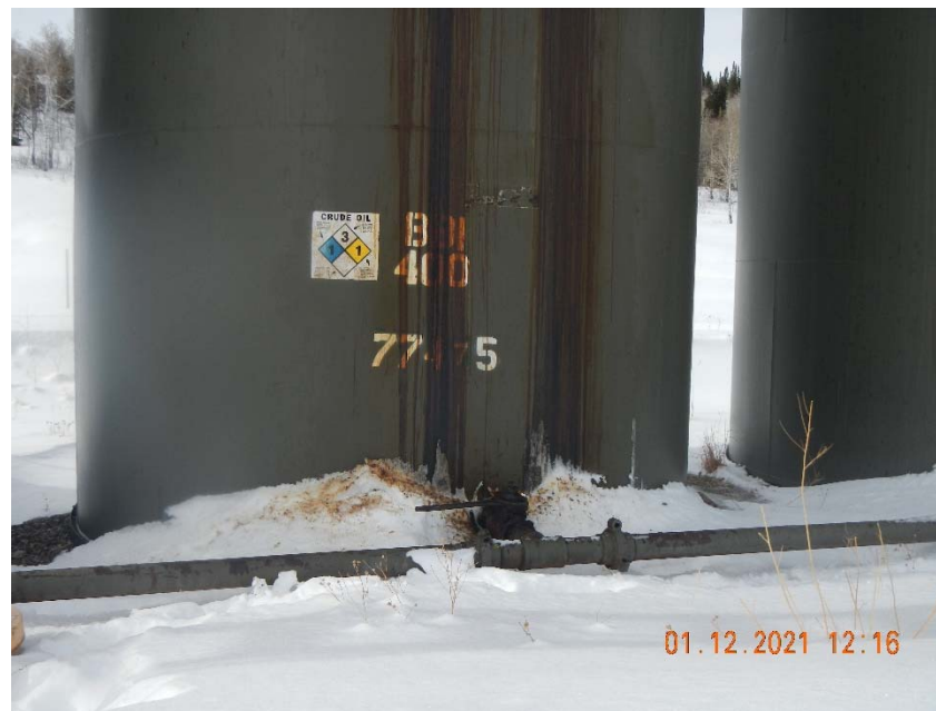
Photo 4. Close-up of staining from apparent overflow.
