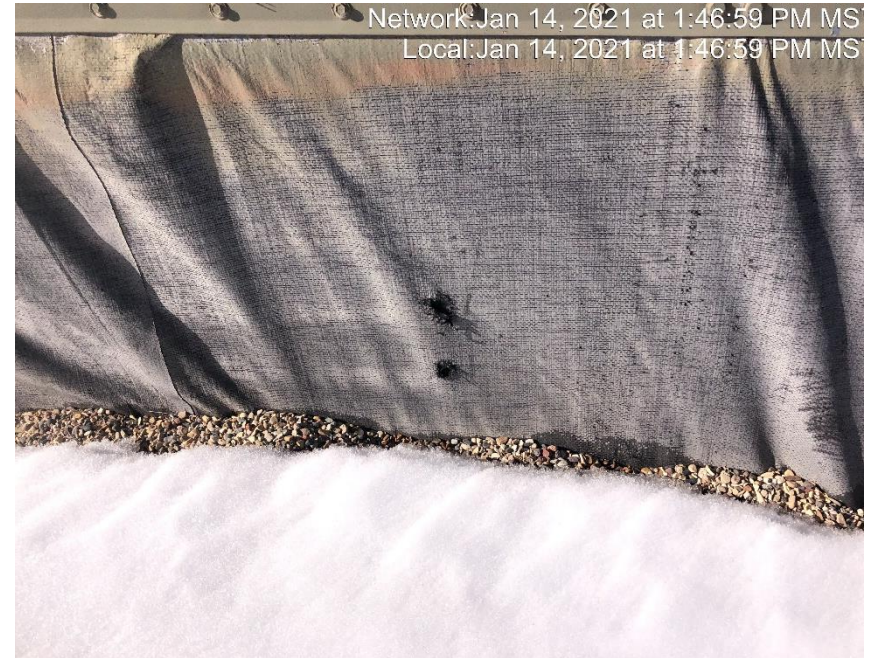
Photo #2638 Multiple holes in tank containment liner.
