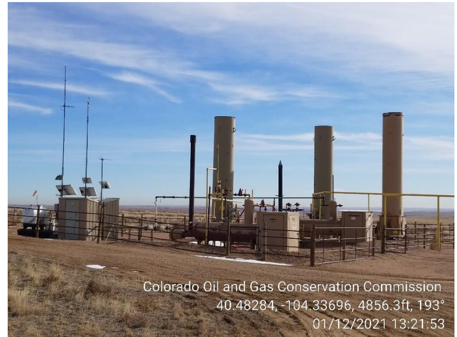
Photo 2 – Separators, ECDS, and Gas Meters
