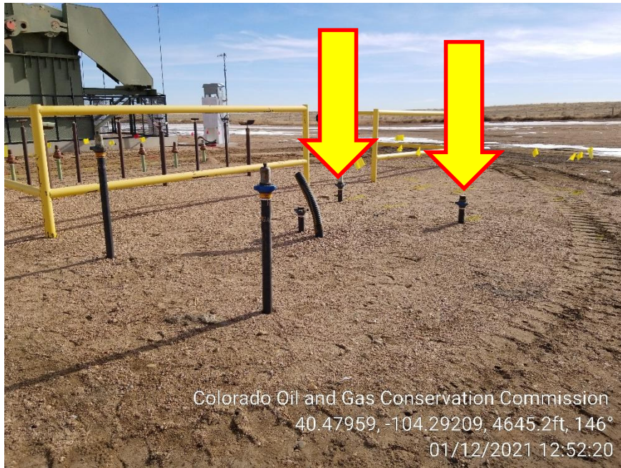
Photo 7 – Unmarked Risers (Marking has faded)
