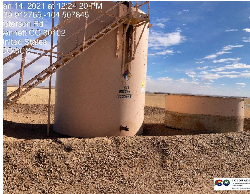
Pic 5 no labels on open top tank
