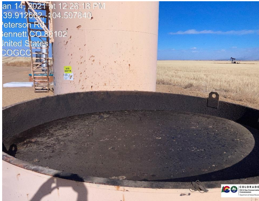
Pic 7 no netting on open top tank / hydrocarbons present
