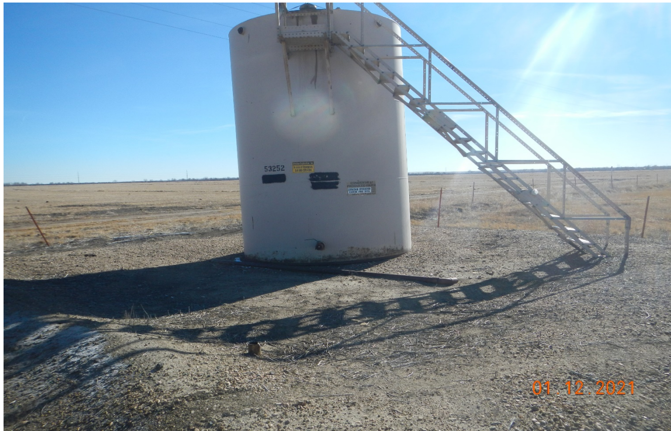
Photo 2. The labeling of the tank is missing information per Rule 210.d.
