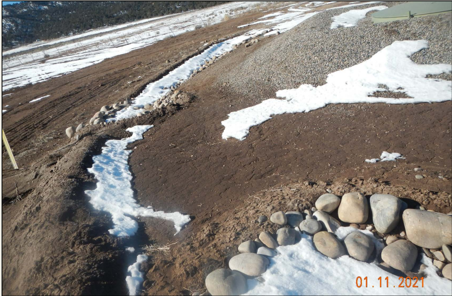
Photo 2. View of the southern project area from the southeastern corner facing westward. Stormwater controls such as berm and cobble lined diversion, are installed and need to be monitored and maintained for function.
