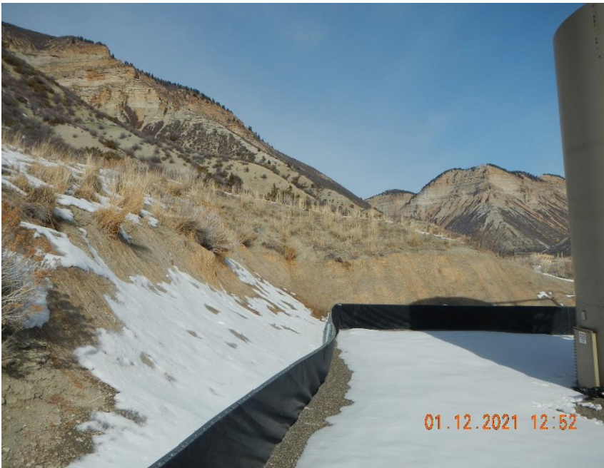
Fissure repaired and Curlex mats installed
