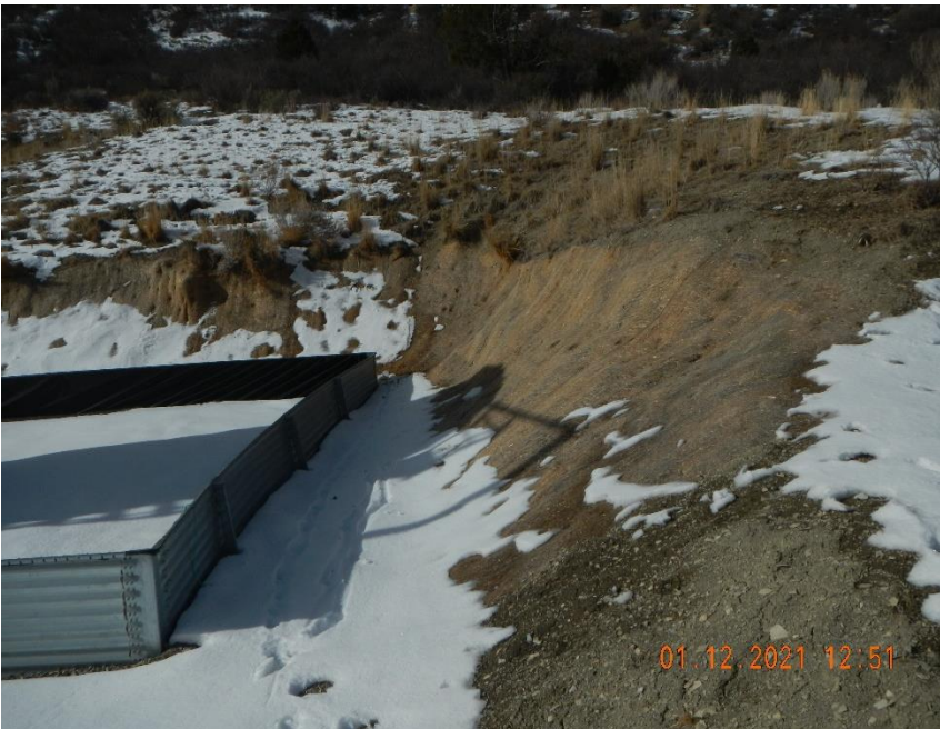
Fissure repaired and Curlex mats installed.
