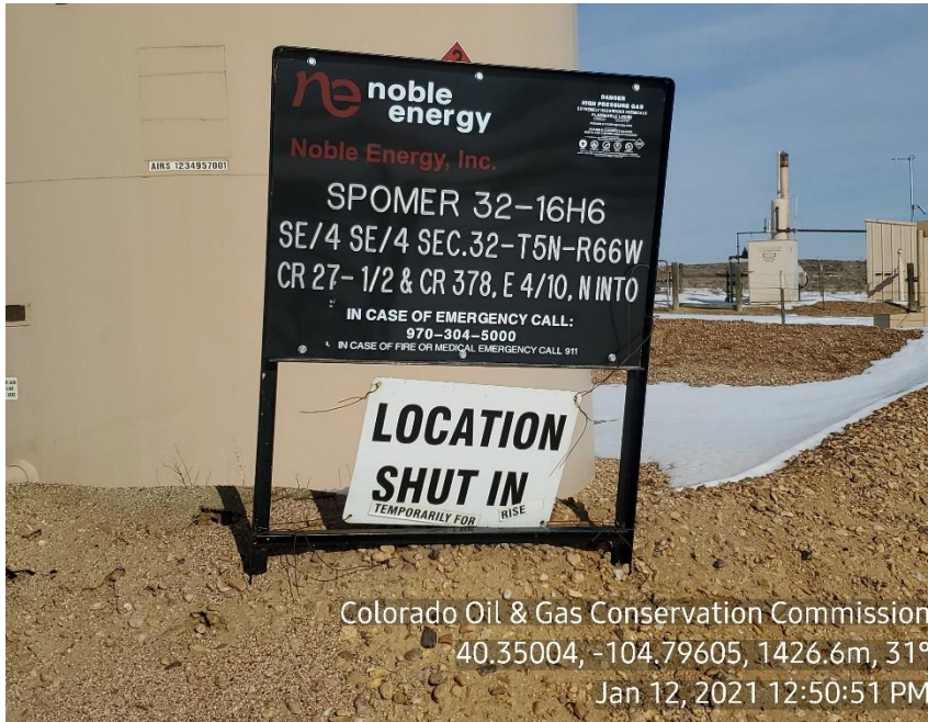
Photo 3: Tank Battery Sign
