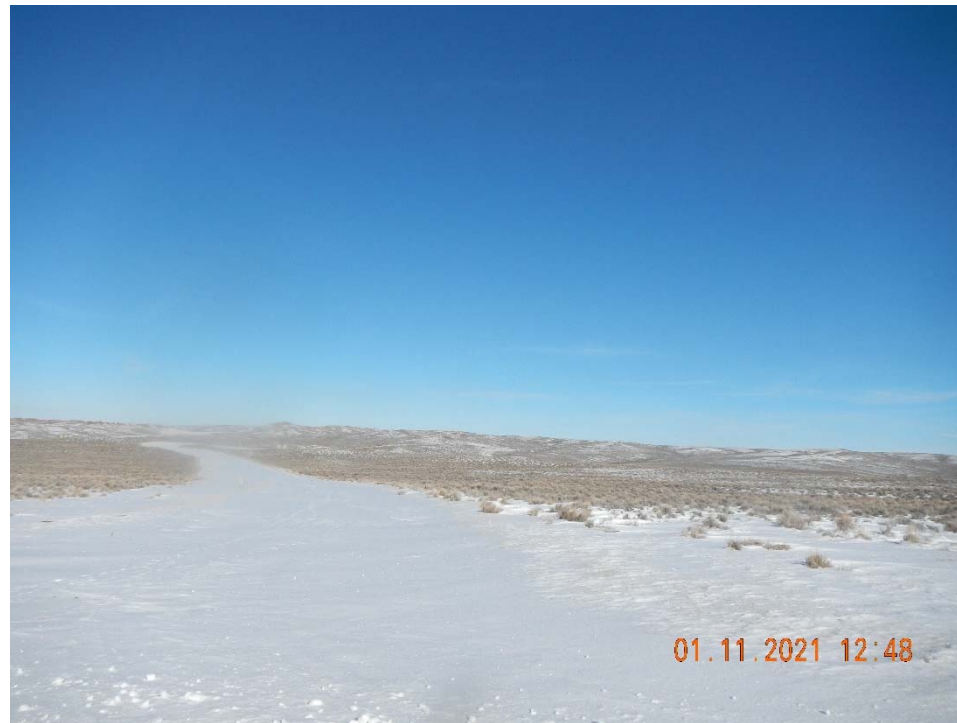
Photo 1. Access road not maintained for winter.
