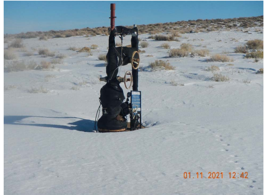
Photo 2. No bradenhead access apparent.
