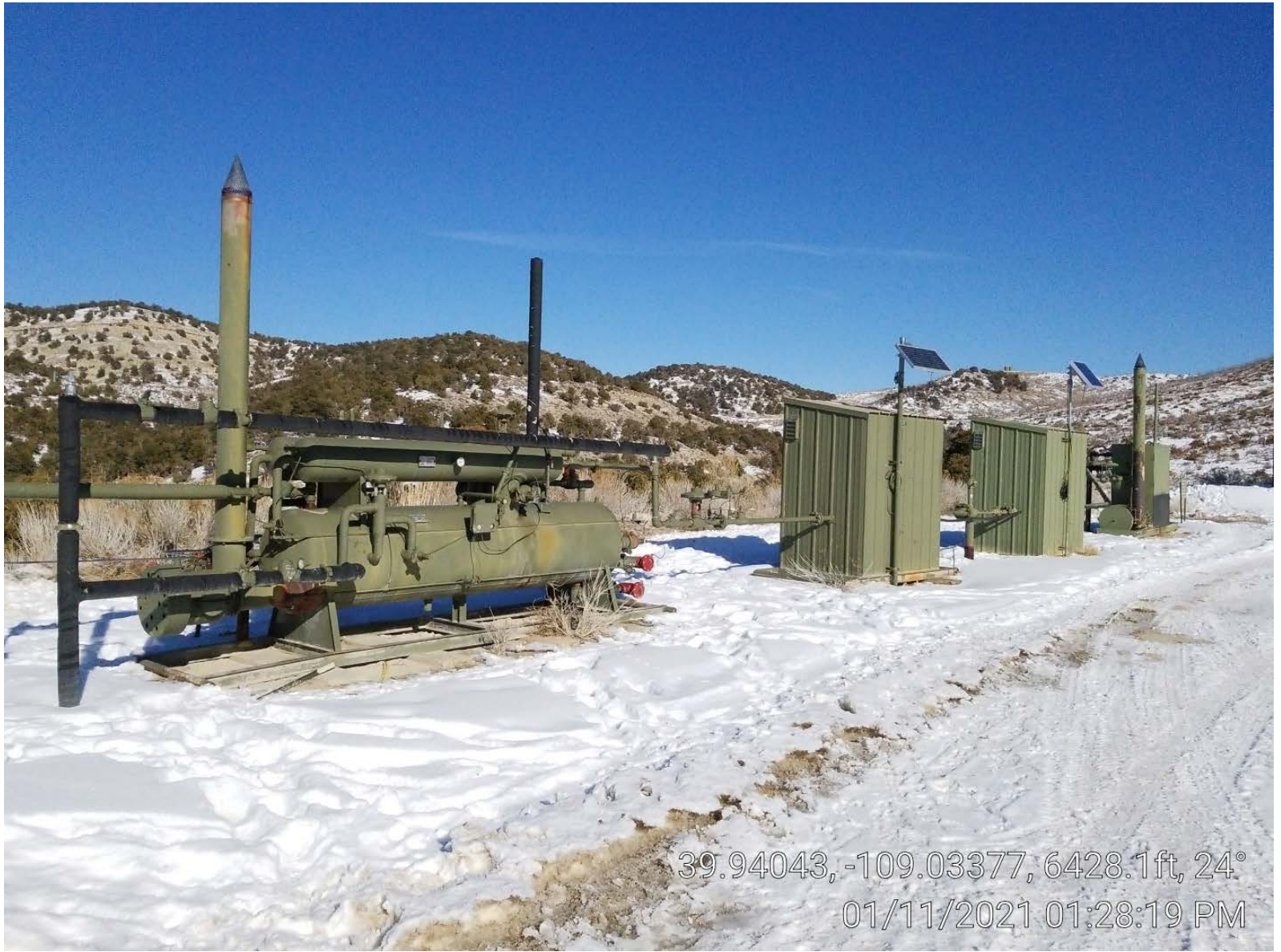
Photo 4. Separators, meter buildings.
