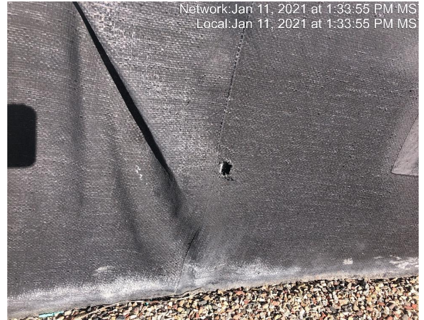
Photo #2600 Multiple holes in tank containment
