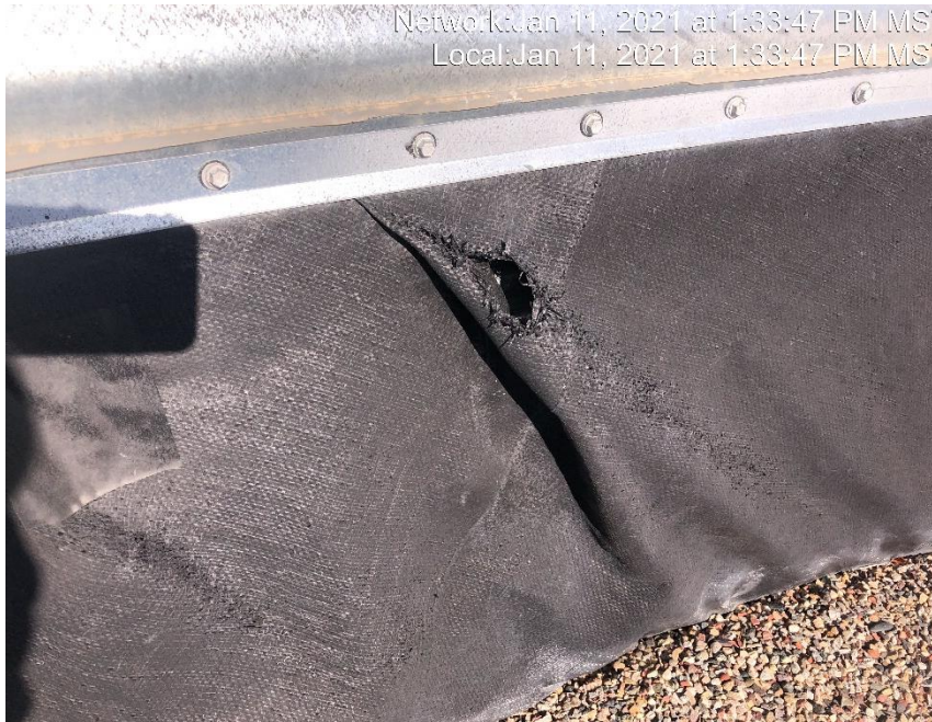
Photo #2599 Multiple holes in tank containment
