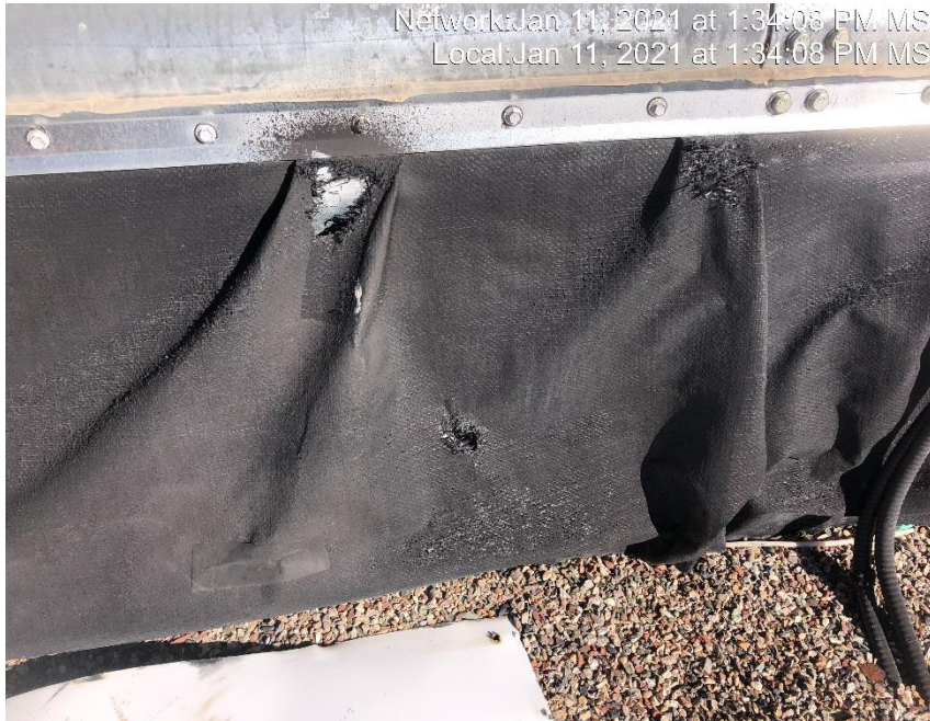
Photo #2601 Multiple holes in tank containment
