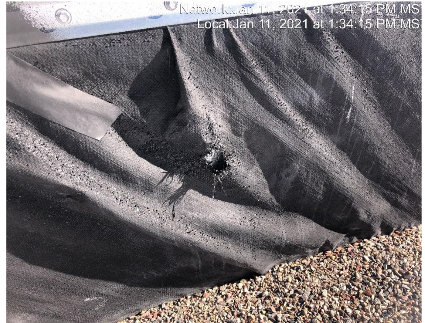
Photo #2602 Multiple holes in tank containment
