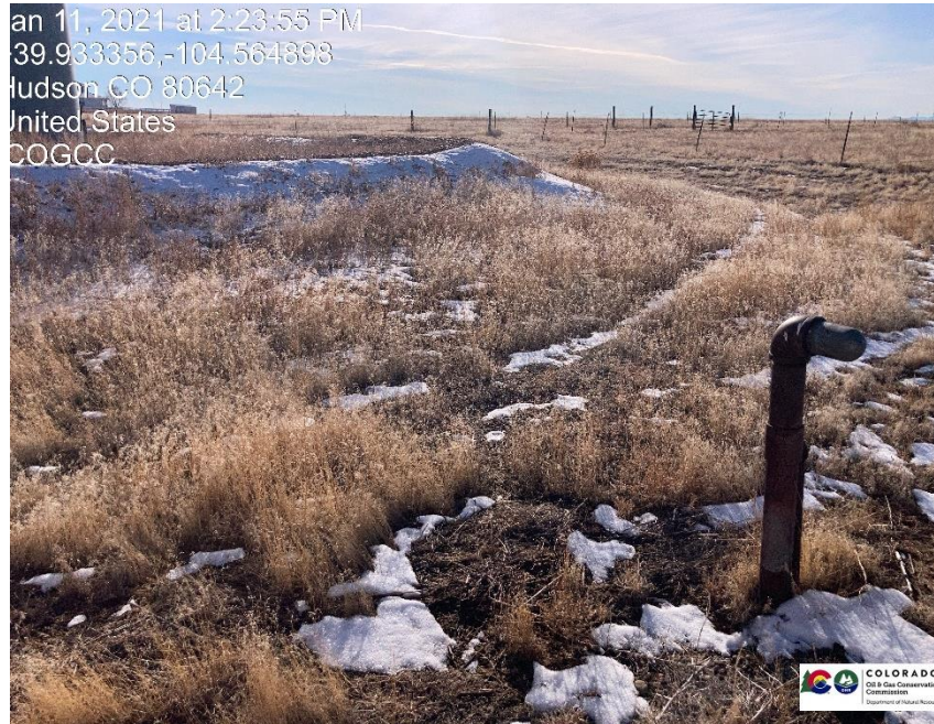
Pic 5 Riser is not IOTO or marked
