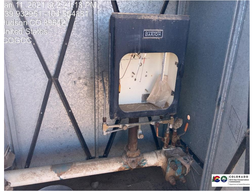
Pic 2 gas meter run unmanaged / no calibration
