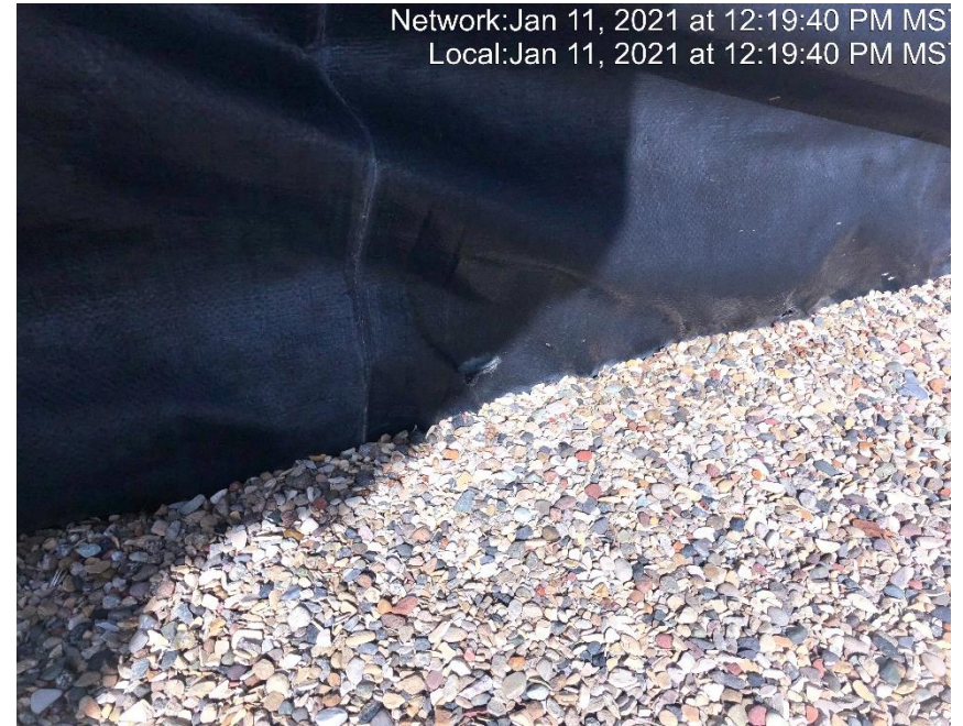
Photo #2594 Multiple holes in tank containment.
