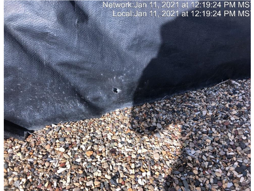
Photo #2592 Multiple holes in tank containment.
