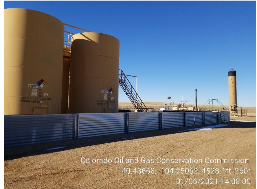
Photo 4 – Tank Battery
