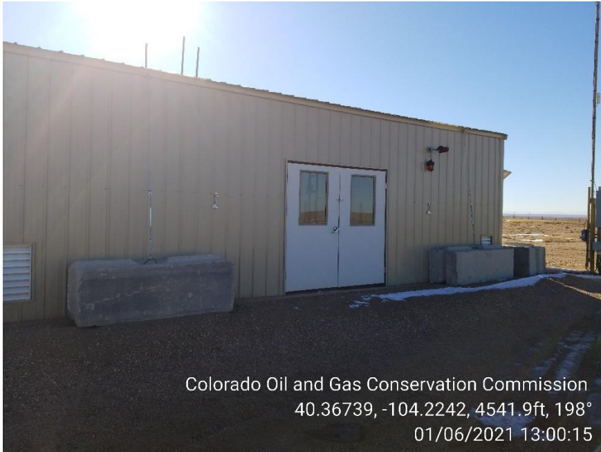
Photo 5 – Gas Lift Meter Shed
